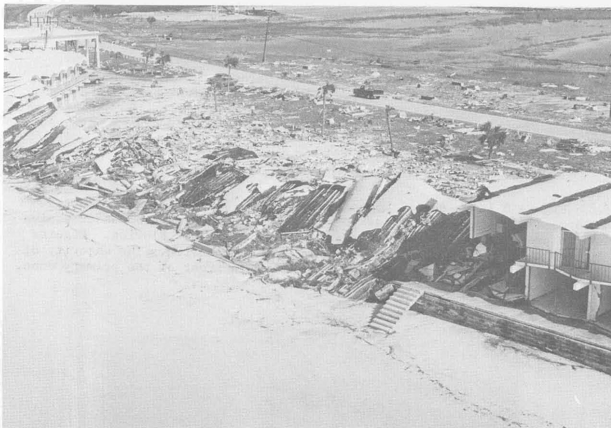
Figure 9 - Storm Damage to the Rountowner Motel
