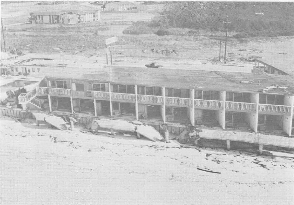
Figure 11 - Typical Damage from Hurricane Eloise
