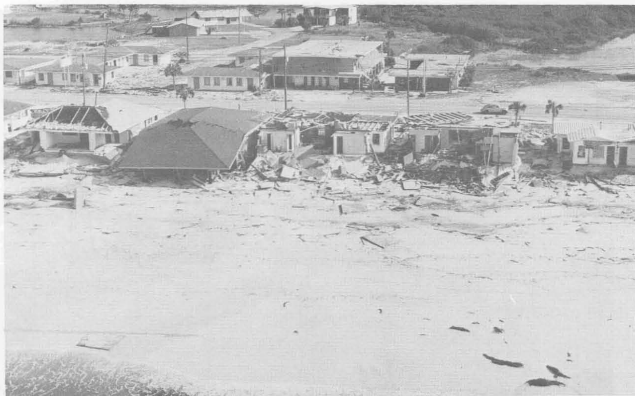
Figure 14 - Typical Damage from Hurricane Eloise
