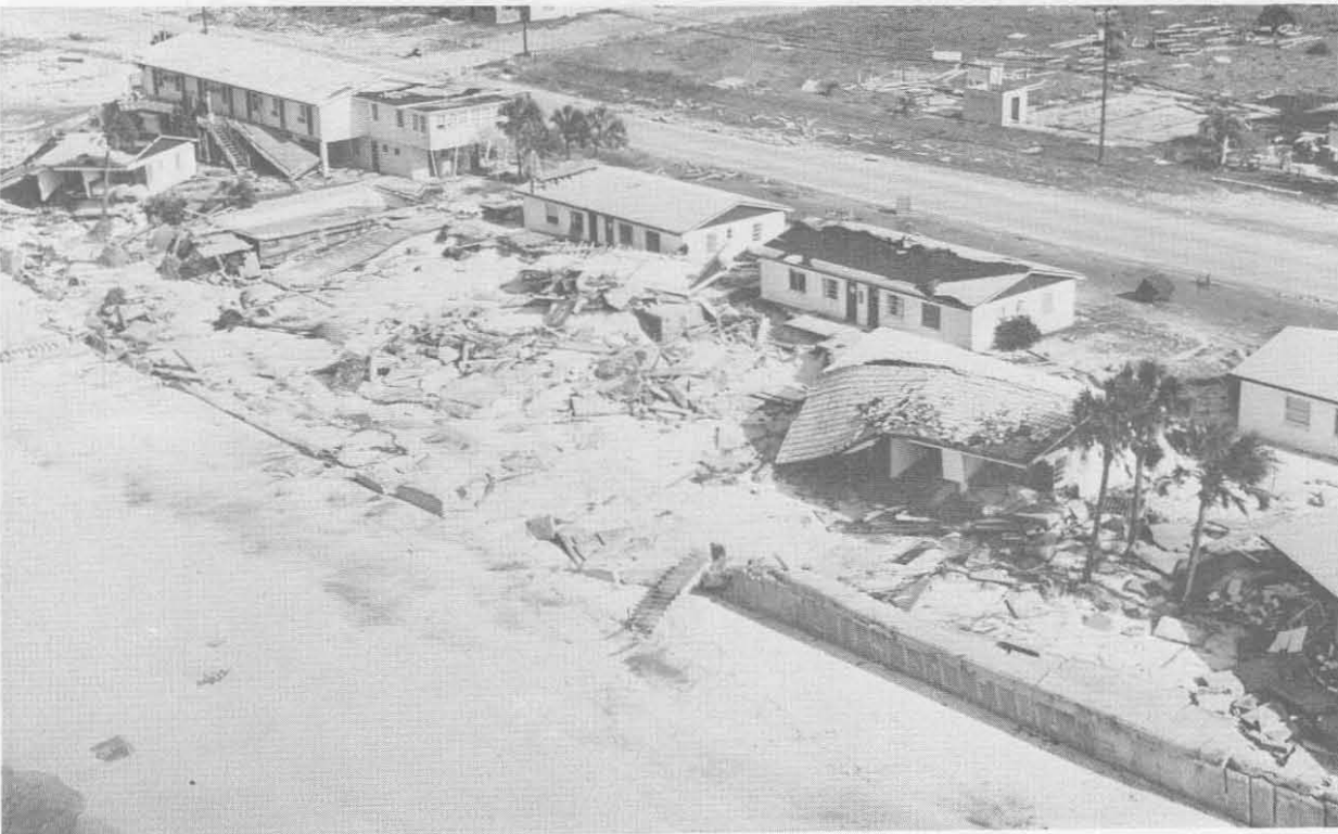
Figure 12 - Typical Damage from Hurricane Eloise
