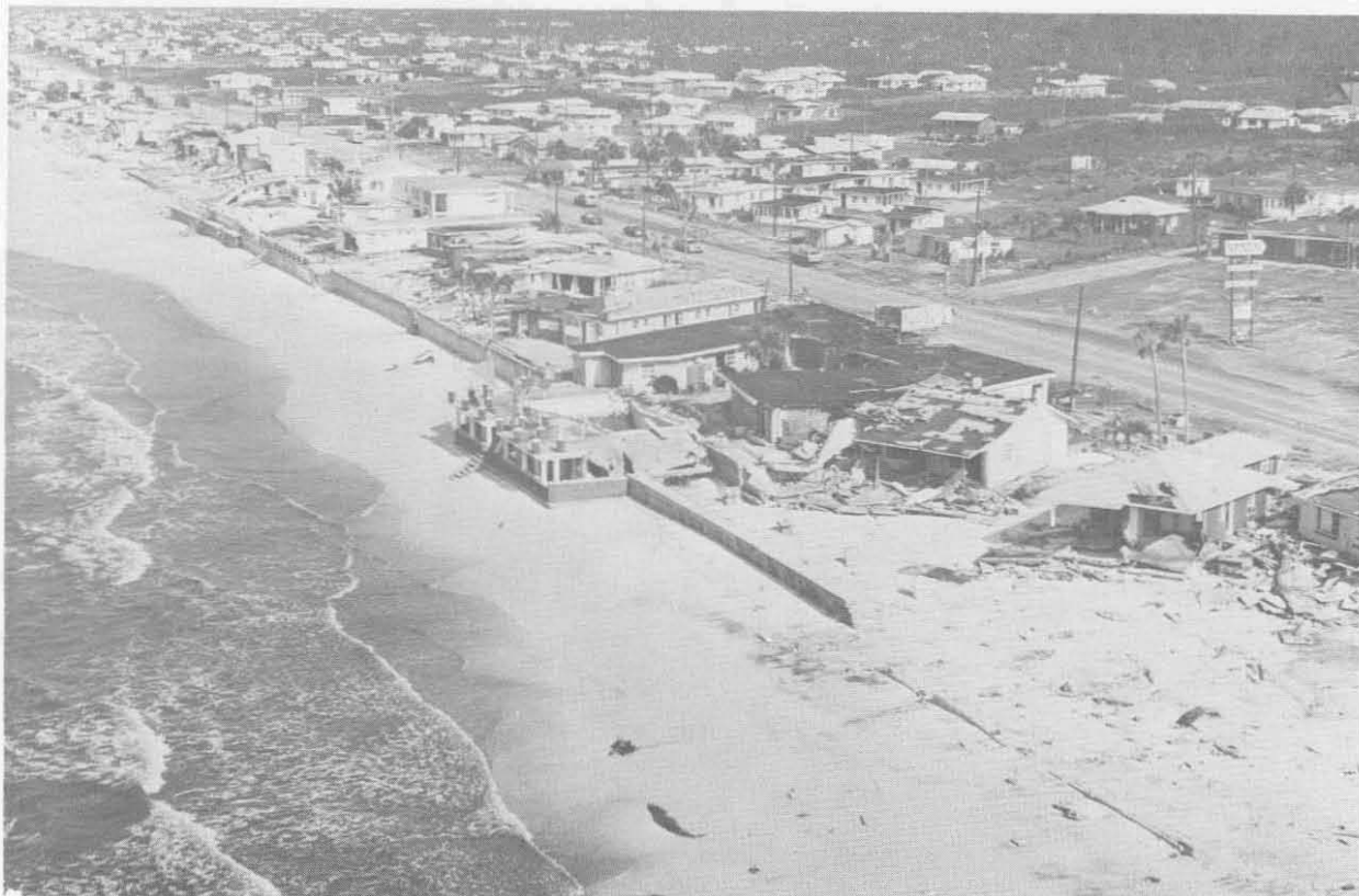
Figure 13 - Typical Damage from Hurricane Eloise
