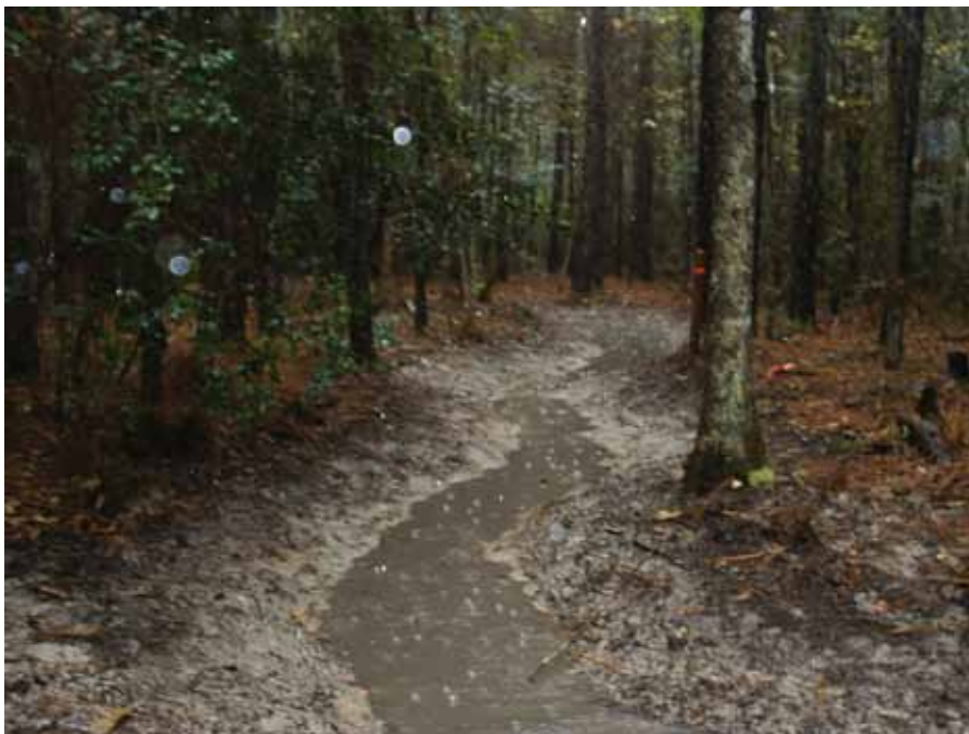
Figure 7. The first rain following channel construction displays the sinuous nature of the constructed stream exhibit.
